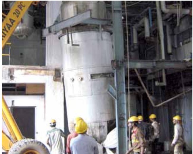
An Enzyme plant shifting on Turn-Key basis : Process reactor being dismantled
